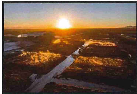
Recology's compost facility in Vernalis covers 120 acres and takes in about 1,500 tons of compostable material daily from San Francisco and elsewhere. The benefits of increased composting are many, but the change won't come cheap.
